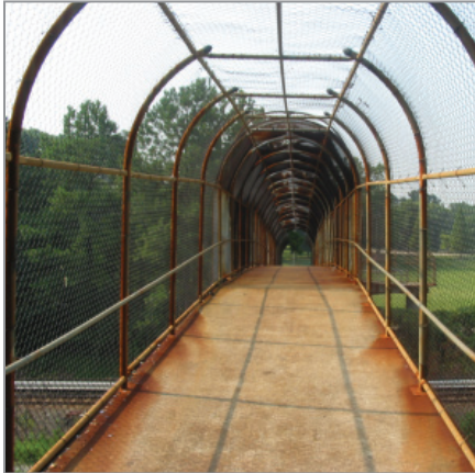
The pedestrian bridge over the railroad tracks is functional, but uninviting
