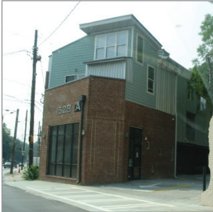
This new mixed-use building was built near the Inman Road and RDA Boulevard intersection
