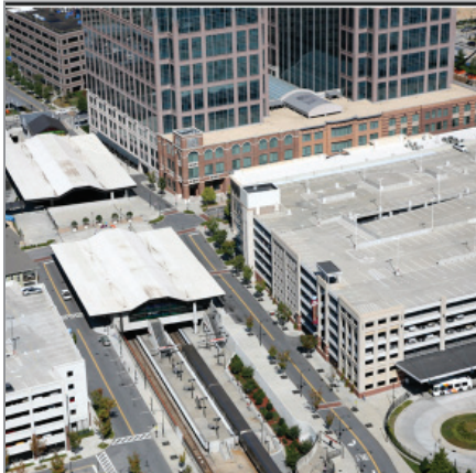
The redevelopment of MARTA's Lindbergh Center Station included parking decks for MARTA patrons
