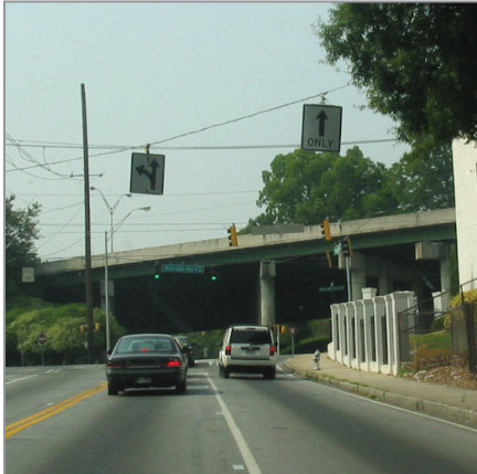
The intersection around I-20 and MLK Jr. Drive must be improved
