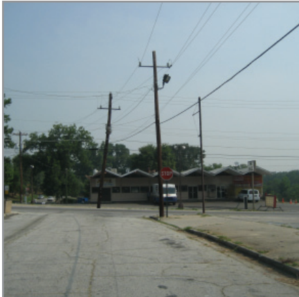
Overhead utilities in the Study Area clutter the sidewalk and disrupt its historic character
