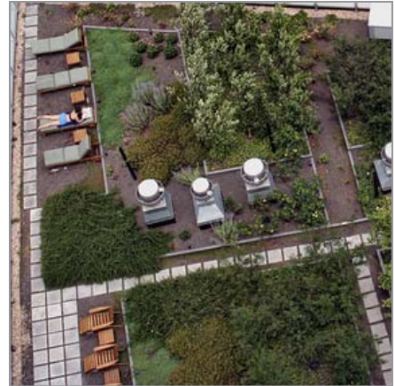
Garden roofs are one strategy to decrease stormwater runoff as the Northside Drive corridor redevelops
