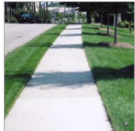
Sidewalk improvements can give a significant facelift to key streets
