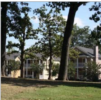
Buildings that face into parks are important for informal security monitoring
