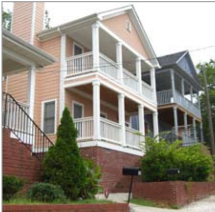
Some infill homes are out of scale with one-story neighboring houses
