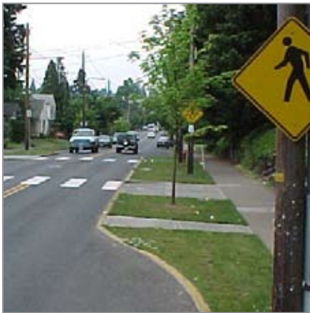
An intersection reconfiguration at Lowery and Mayson Turner could provide additional greenspace
