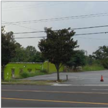
Parking lots along Northside Drive contribute to litter and stormwater runoff
