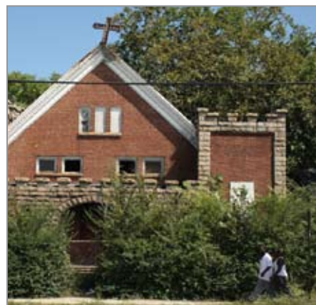
Abandoned buildings could be renovated to avoid further deterioration
