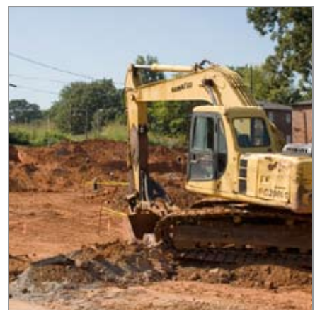
Construction of the new Vine City Park is now complete
