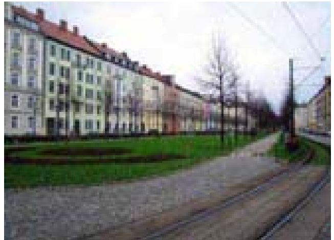
In many highly livable European cities, building height corresponds to the width of the adjacent public space
