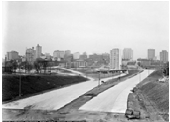
Construction of what is now Freedom Parkway began in 1964 and resulted in the demolition of many buildings (Image courtesy Special Collections and Archives, GSU)
