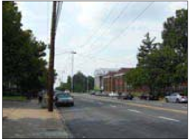
Boulevard as it is today, with utility poles, little greenery, and dangerous pedestrian crossings
