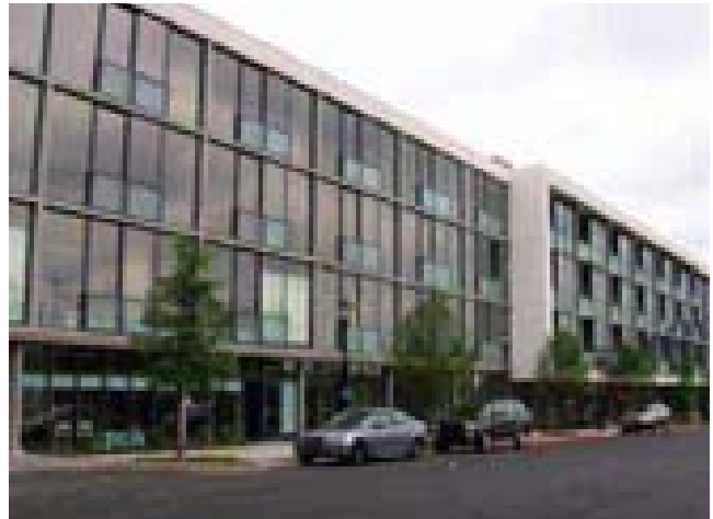
Mixed use developments such as this one will form an important part of the future land use mix in the study area
