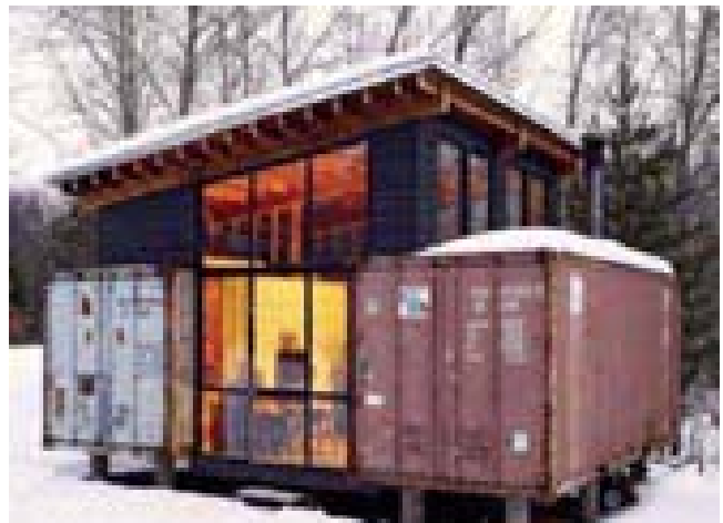
One example of a temporary workspace structure made from recovered shipping containers
