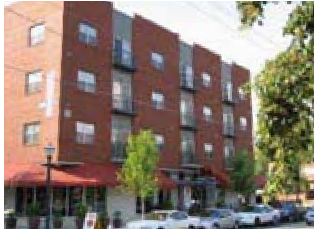
In the Old Fourth Ward, the entire neighborhood will be mixed-use, as well as individual buildings
