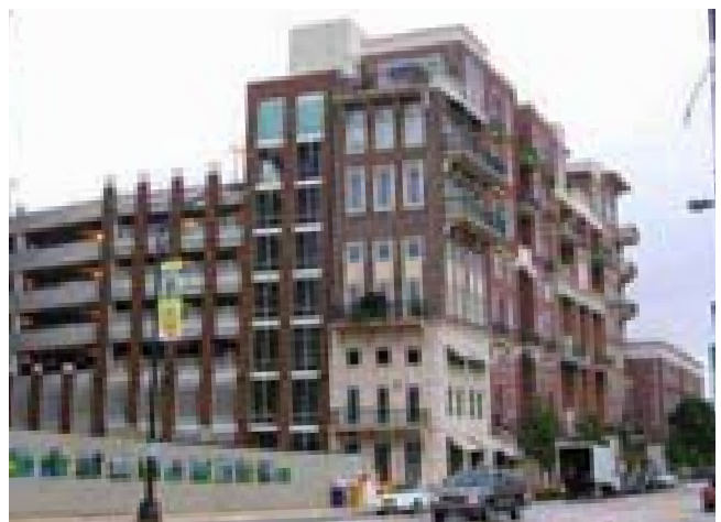
This photo shows how "liner" uses can screen a parking deck from the street; when a building is built on the adjacent vacant lot the parking will be completely unseen
