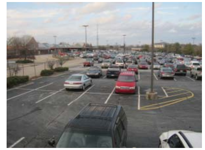
East Point MARTA Station parking lot is relatively full during the weekday
