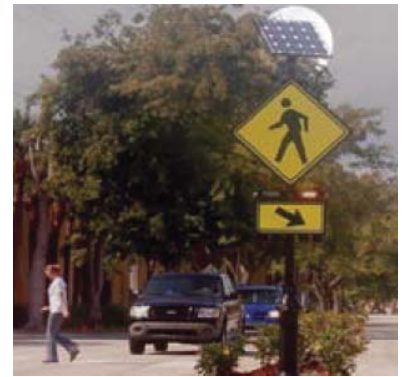
Activated, solar-powered RRFB at an unsignalized intersection flash using an irregular flash pattern (Source: FHWA)
