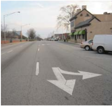
Main Street downtown at the East Point MARTA station lacks defined streetscaping
