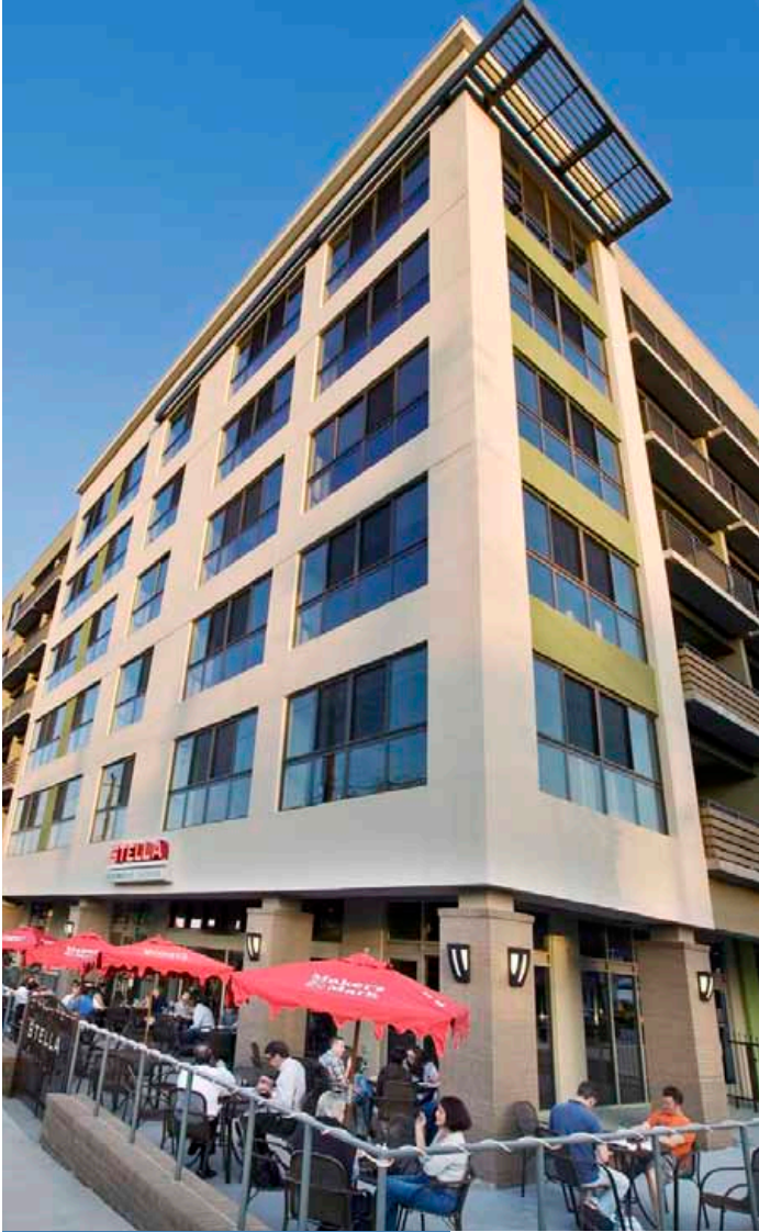
The LEED-Certified Oakland Park Mixed-Use Development is a good example of sustainable development within the Downtown area.
