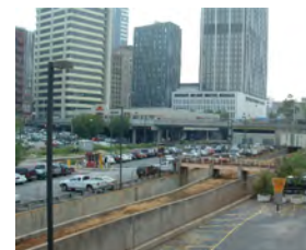
Railroad Gulch Looking East
