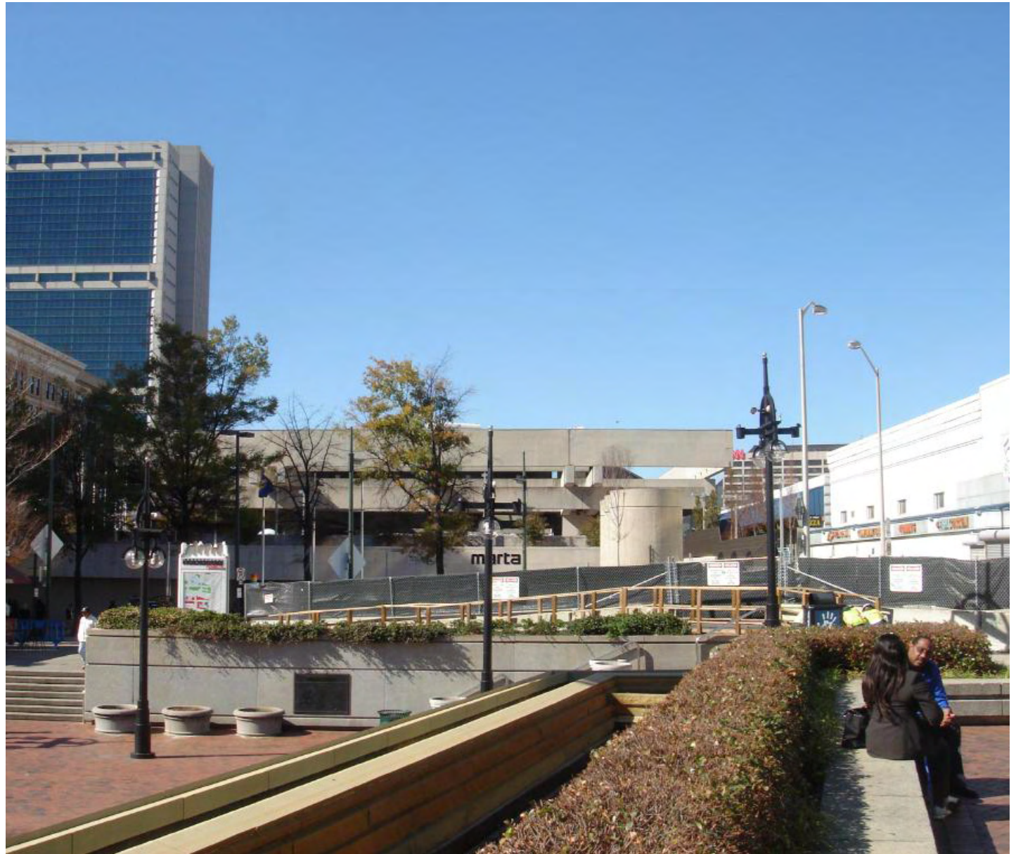
The current Five Points MARTA station is both a literal and figurative barrier between the North-South and East-West corridors. A public plaza and a sense of transparency will help reestablish this nexus of our city.
