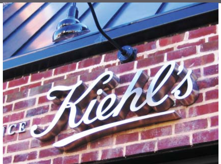
EXTERNALLY ILLUMINATED SIGNAGE A more traditionally-inspired sign with lettering or logos lighted by fixtures mounted to the wall.
