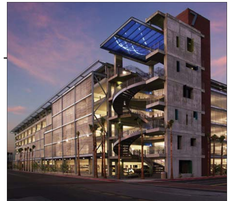
While there is parallel parking on the street and some surface parking, the majority of parking in the district is handled by multi-story garages.
