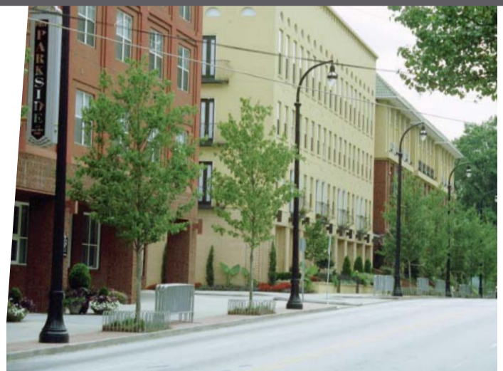
PARKING STRUCTURE FENESTRATION The large yellow building in the center of this image is a parking garage with a 40' liner of residential at the frontage.
