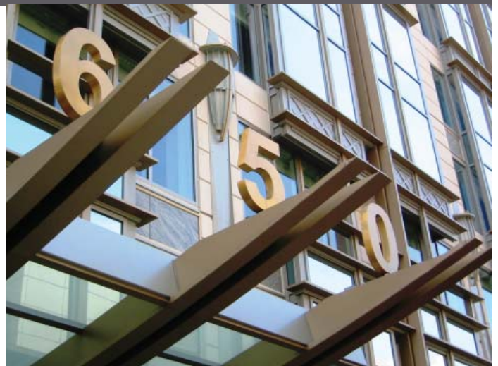
CANOPY LETTERING Larger buildings may be identified by street number - which may be attached directly to the lobby canopy.
