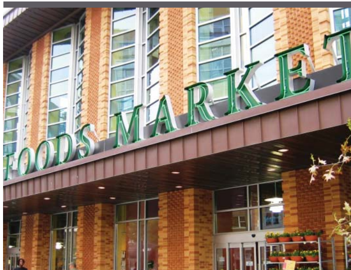
INTERNALLY ILLUMINATED SIGNAGE Channel letters made of metal, internally lit with neon tubes.
