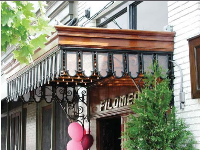
CANOPY STRUCTURE AND MATERIALS Metal support chains, wood and glass combine to provide shelter over the entrance to a restaurant. This canopy is also lighted underneath.
