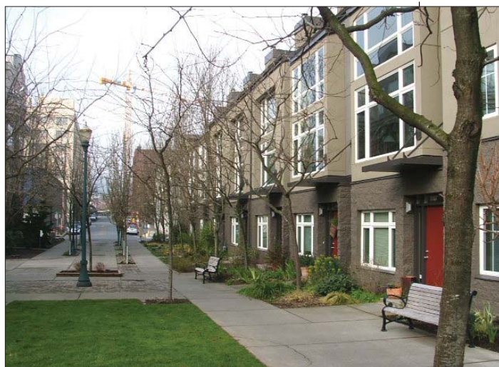
The townhomes help transition from higher density residential in the Science and Technology Center to single family homes in the neighborhood.
