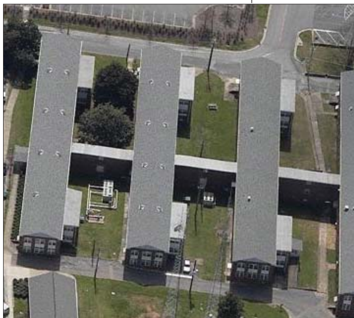
Office and Administrative uses will occupy Buildings 128, 129, 130, and 131.
