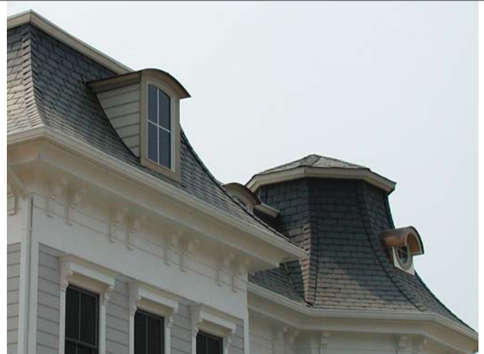
OTHER ROOF SHAPES Turrets, domes, and other roof shapes may be permitted, provided they are sized correctly, and used at appropriate locations.
