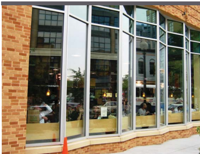
GROUND LEVEL STOREFRONT EXPRESSION Larger buildings with retail space in the ground floor
