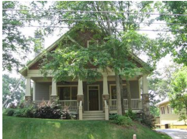
Example of New Infill Housing in Edgewood
