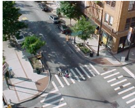
Sidewalk extensions, or bulbouts, provide traffic calming at the major intersections of Whitefoord
