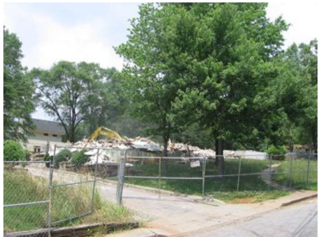
Edgewood Housing Units - Post-Demolition
