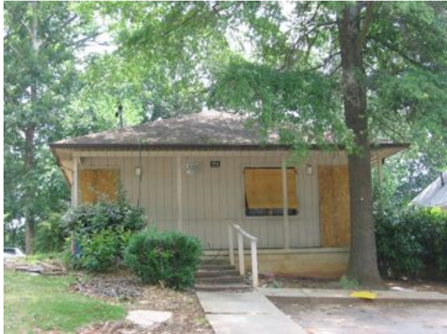
Edgewood Housing Units - Pre-Demolition
