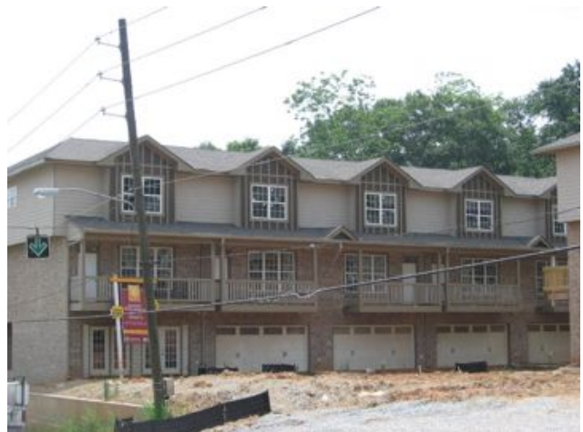
Townhomes Under Construction along Memorial Drive
