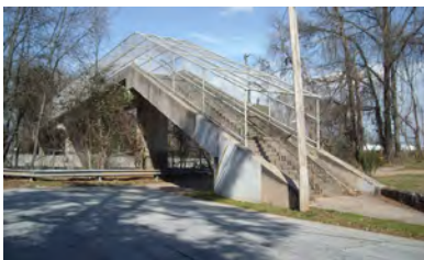
Pedestrian Bridge over Langford Parkway connects the Colonial Hills neighborhood
