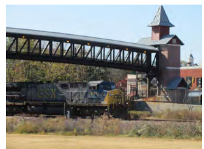
The pedestrian bridge across the MARTA and freight rail lines in downtown
