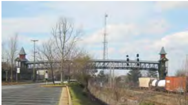
Pedestrian Bridge near the East Point MARTA Station is an iconic feature in the downtown
