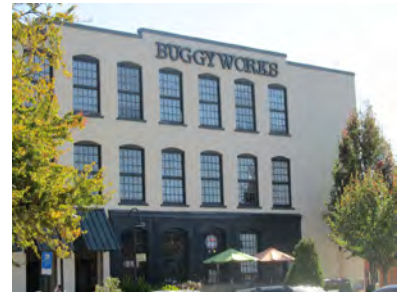
Previous adaptive reuse within the study area
