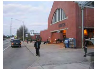
East Point MARTA Station entrance improvements are needed for safety and aesthetics
