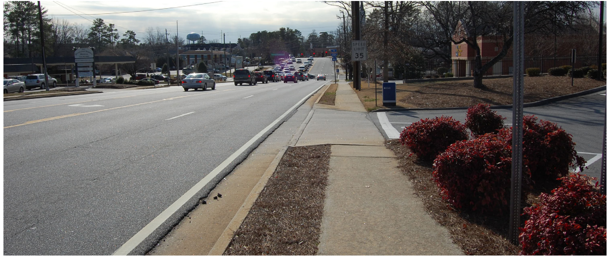
Sidewalk along Mount Vernon Road
