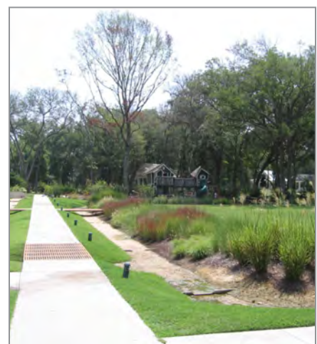
Roadside swales and infiltration can be visually pleasing and reduce water erosion
