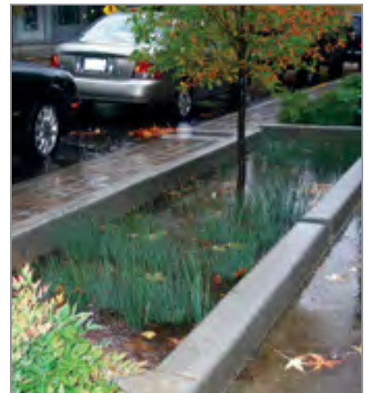
Curbside bio-swales could improve water quality
