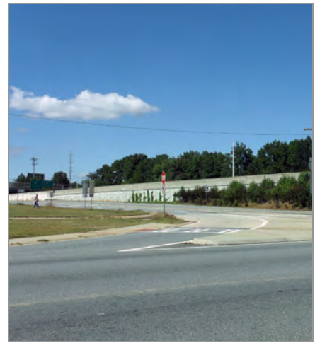
The Buford Highway and I-285 interchange is a key facility
