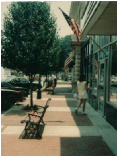
Significant streetscape upgrades are recommended for the entire LCI area.
