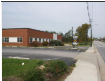
The adaptive reuse of industrial buildings is ushering in new residential growth.
