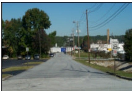
The current condition of east-west connections: no pedestrian facilities present.
