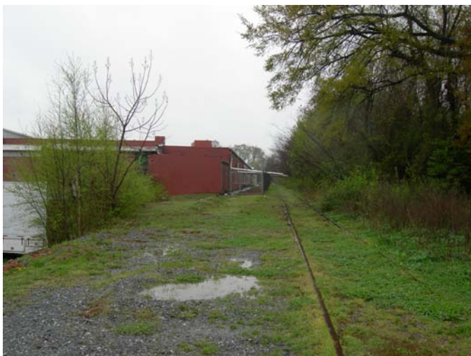
Potential areas in which buildings have encroached into the BeltLine right of way over time will need to be dealt with on a parcel by parcel basis.
