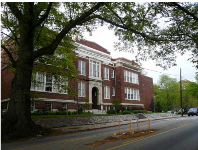
The Highland School Lofts is a converted school listed on the National Register of Historic Buildings
