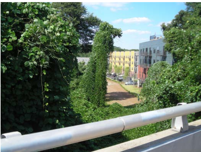
Highland Avenue crosses over the BeltLine right-of-way. Picture shows bridge guardrail in foreground. New development and the overgrown right-of-way shown under the bridge
