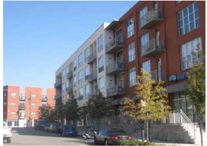
New mixed use development will put people and jobs within walking distance of transit.
