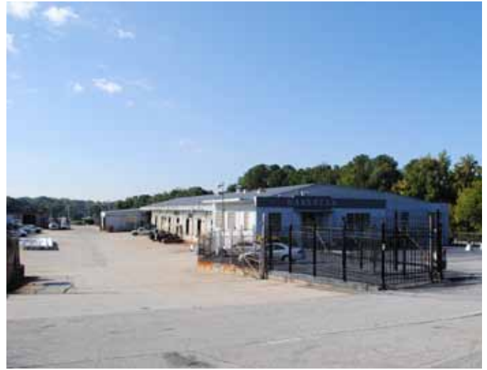
A flexible planning approach should preserve active industrial businesses today while allowing future opportunities for mixed use redevelopment.
