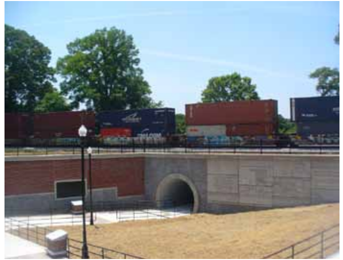
This pedestrian underpass in downtown Kennesaw is an example of a bicycle and pedestrian underpass that can be used to pass under rail lines in the subarea.
