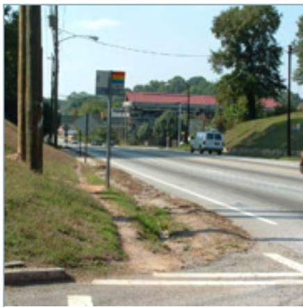
Missing sidewalks prevent patrons from safely accessing bus and rail transit in the Study Area
