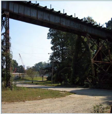
This trestle over North Avenue provides one of the few east-west street connections in the Study Area
