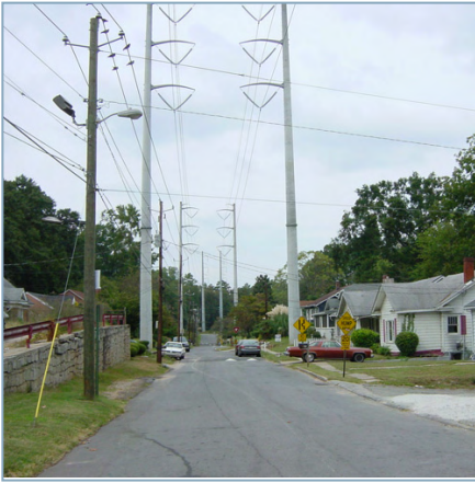
Major utility lines run down the middle of Florence Place and disrupt its residential character
