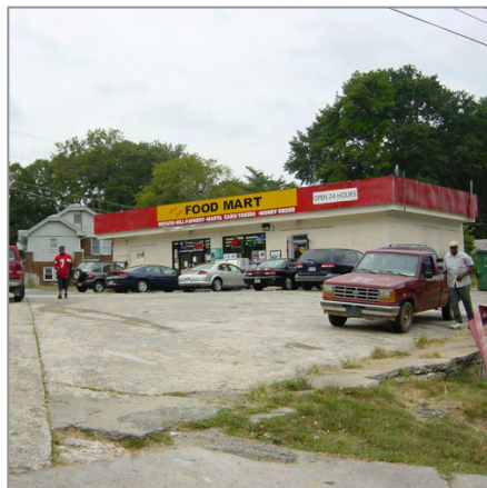
This business represents the highway oriented commercial uses lining Donald L. Hollowell Parkway
