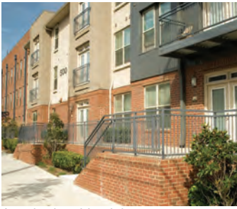
Attached residential Photo Source: TSW
