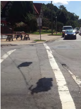
Some crosswalks on US 278 have inadequate striping.
