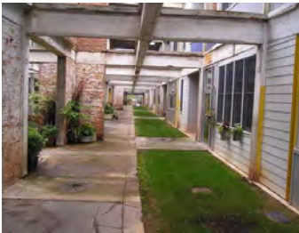
Conversion of former warehouse into retail and condo space
