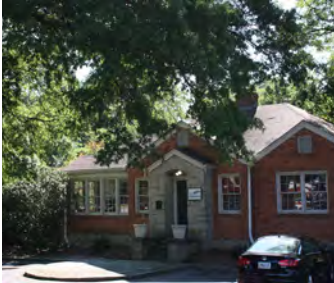
Existing adaptively reused cottage on North Clarendon Avenue
