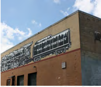
Existing warehouse building in Rail Arts District
