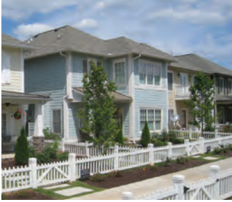
Low-scale building forms appropriate in the Northern Gateway Photo Source: TSW
