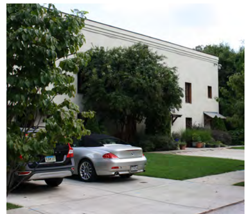
Multifamily Residential: new townhouses
