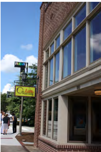
Hairston Building in Main Street Vernacular style
