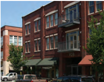
Potential scale for redevelopment on MARTA property Photo Source: TSW
