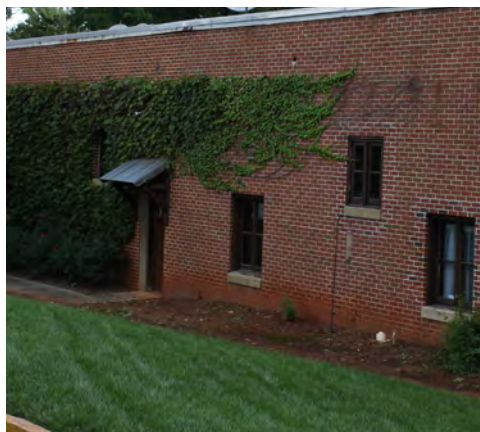
Multifamily Residential: condominiums in a former warehouse
