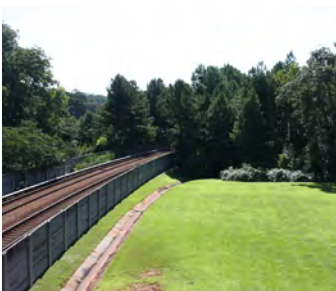
MARTA rail and adjacent greenspace east of North Clarendon Ave
